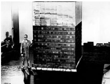
One of at least 29 experimental piles that were constructed in 1942 under the West Stands of Stagg Field. Each tested elements incorporated into the final design.
